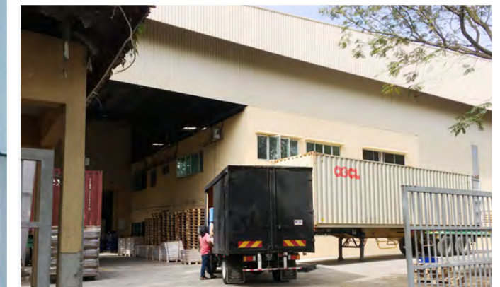
With the Group's tremendous growth, our production facilities have simultaneously grown to support the ever-increasing demand of our products.
